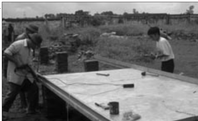
Construction of the tunnel dryer
